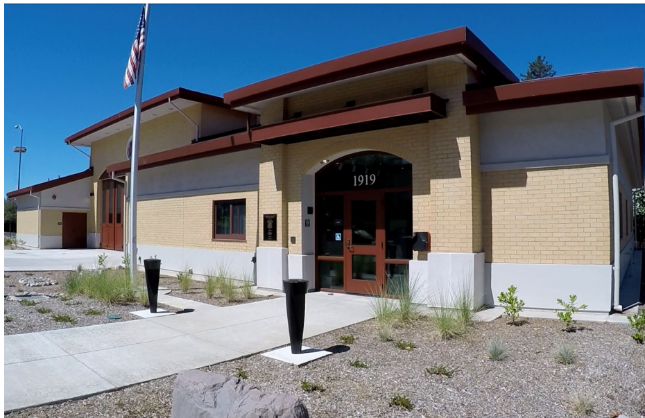
Figure 1-3 Fire Station No. 9
