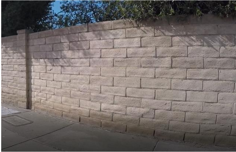
Figure 1-7 Wall Material: Slump Block
