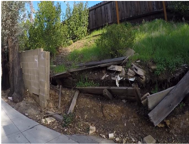
Figure 1-15 Wall Condition 5 Example
