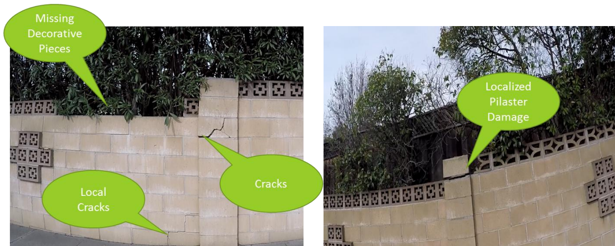
Figure 1-17 Wall Repair Example
