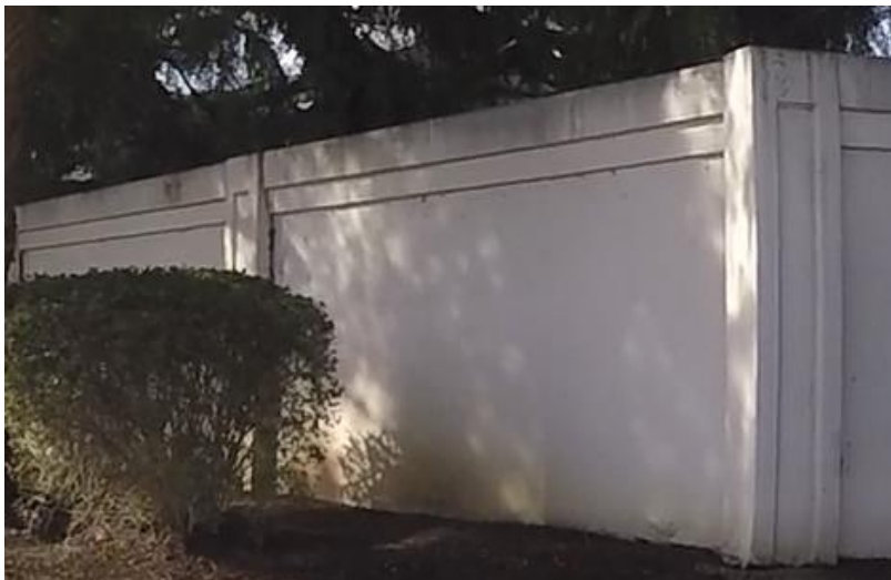
Figure 1-6 Wall Material: Concrete Panel (Pre-Cast)
