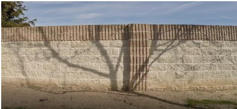
Figure 1-5 Wall Material: Concrete Block (New Style)
