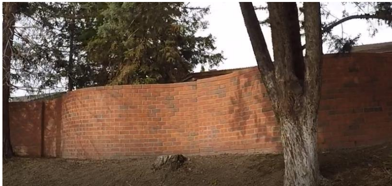
Figure 1-3 Wall Material: Brick
