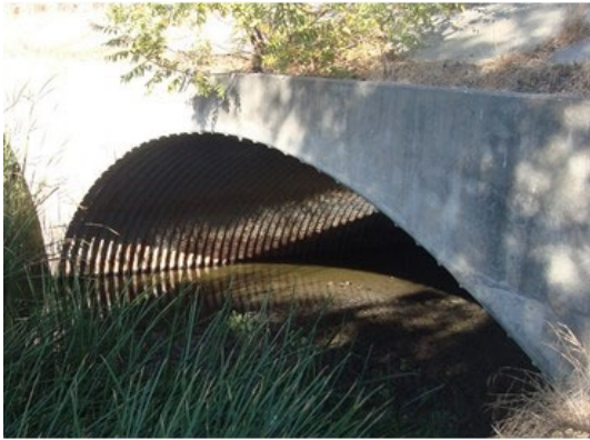
Figure 1-8 Substructure – Culvert
