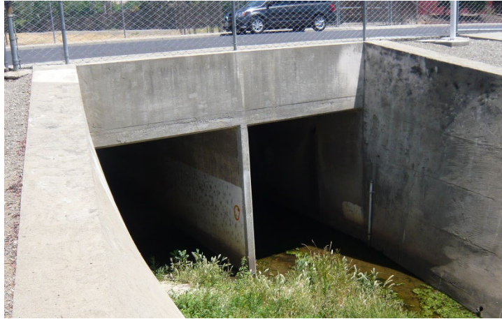
Figure 1-2 Vehicle Bridge - Culvert
