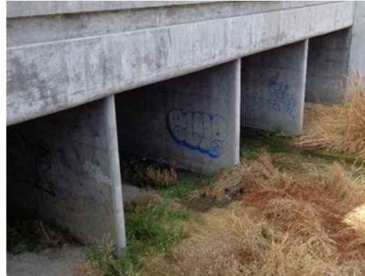
Figure 1-8 Substructure – Culvert
