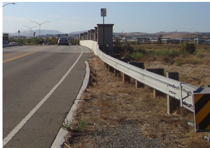
Figure 1-10 Superstructure – Guardrail
