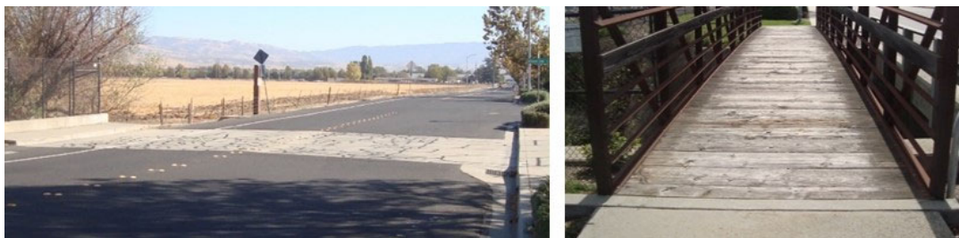
Figure 1-7 Superstructure – Deck
