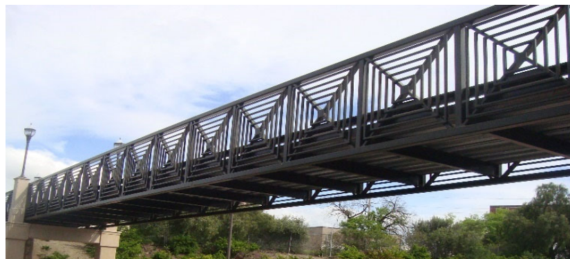
Figure 1-9 Superstructure – Truss
