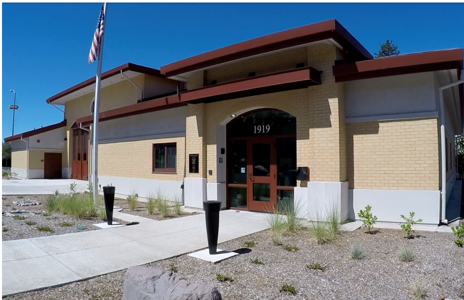
Figure 1-3 Fire Station No. 9
