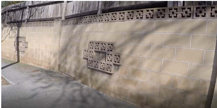
Concrete Blocks (Old Style)
